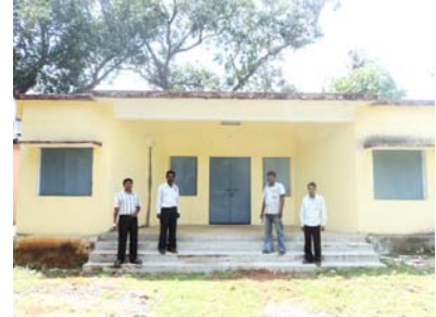
Idle DDL building at paralakhemundi
