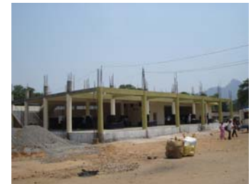
Incomplete bus terminus at Rayagada
